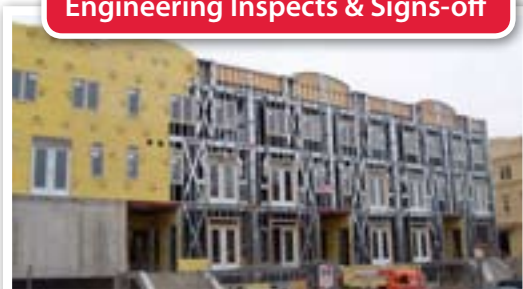
Engineering Inspects & Signs-off
